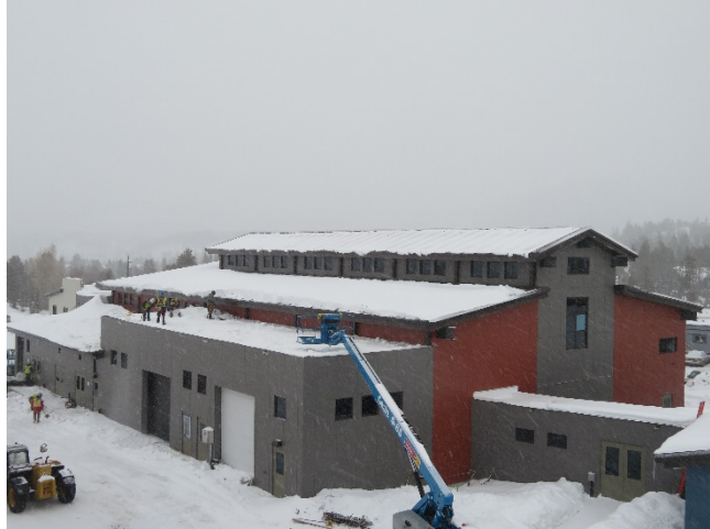
02/19/2020 – MTB Removing Snow From Roof
