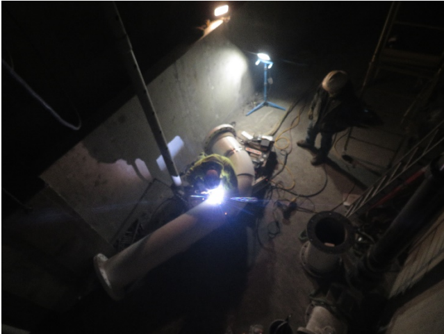
02/05/2020 – Finished Water Pump Station Pipe Fitting
