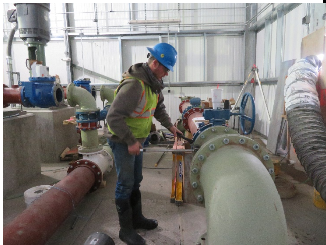
02/24/2020 – Finished water Pump Station Torqueing Bolts
