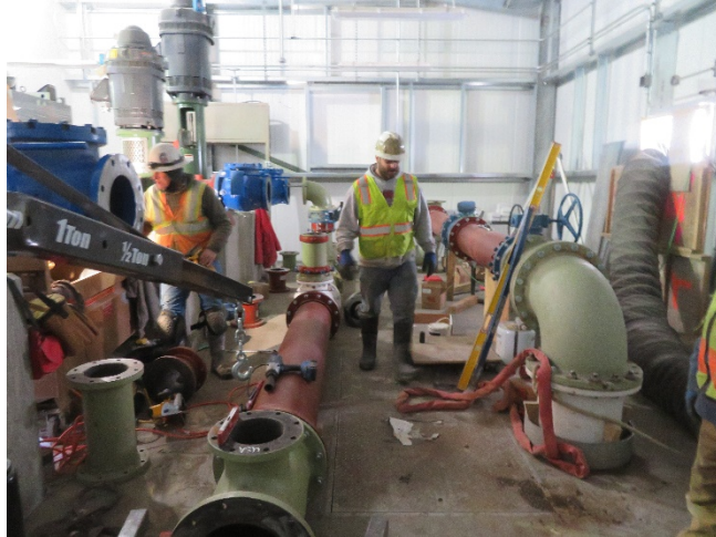
02/12/2020 - Raw Water Pump Station Process Piping
