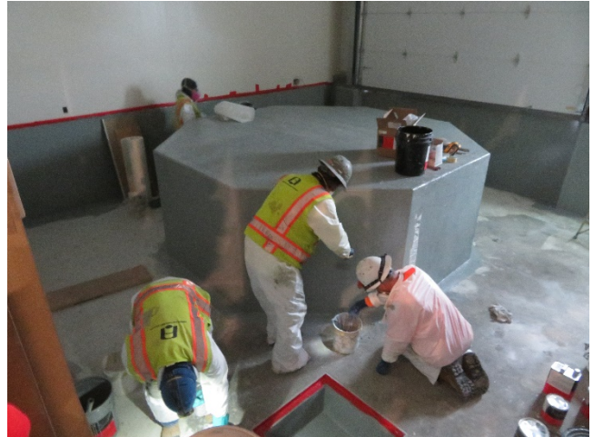
02/06/2020 – PACL Room Fiberglass and Epoxy
