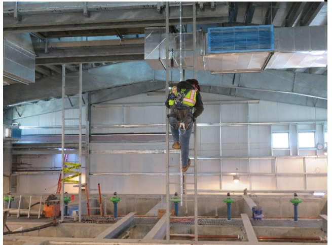
02/11/2020 – MTB HVAC Unit Access Ladder
