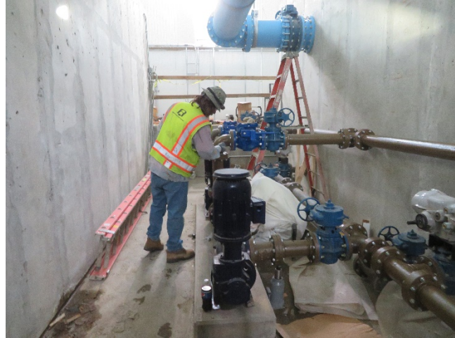
01/17/2020 – MTB Sedimentation Basin Settled Sludge Piping Painting
