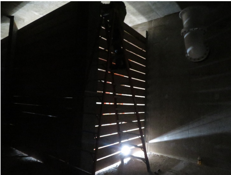
Clearwell 1 Baffle Wall 01/29/2020
