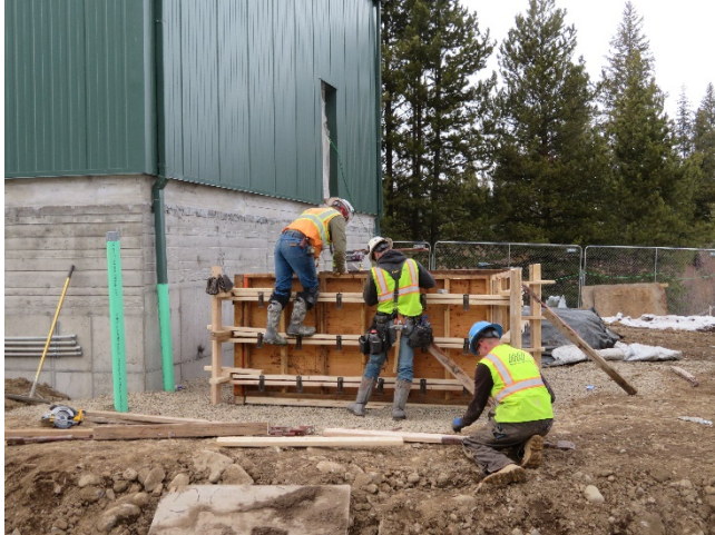
01/16/2020 - Raw Water Pump Station Surge Tank Slab on Grade
