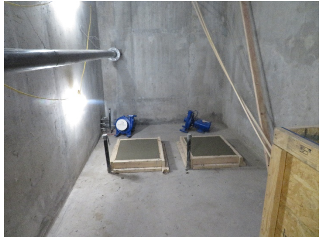
01/10/2020 – Residuals Recycle Pumps Equipment Pads
