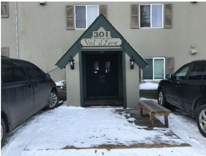
Figure 3: Existing open air entry
