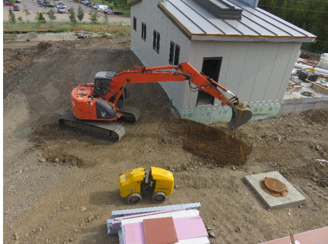
8/29/2019 – Finished Water Pump Station Backfill
