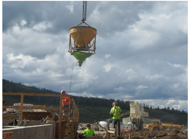
8/08/2019 – Residuals TARN Pipe Encasement
