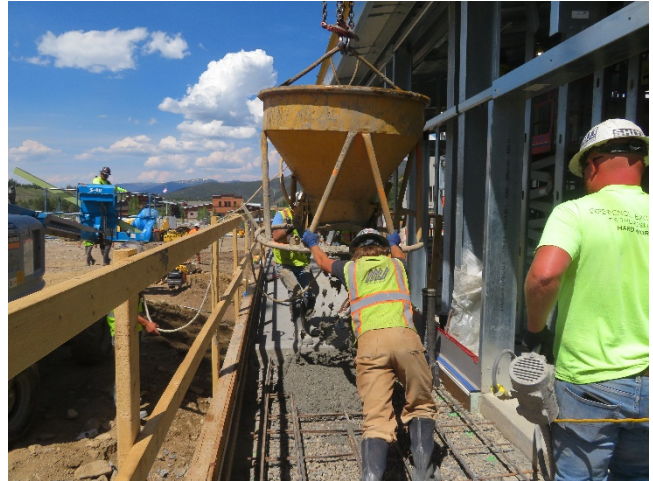
8/06/2019 – MTB Exterior Sidewalk Concrete Placing
