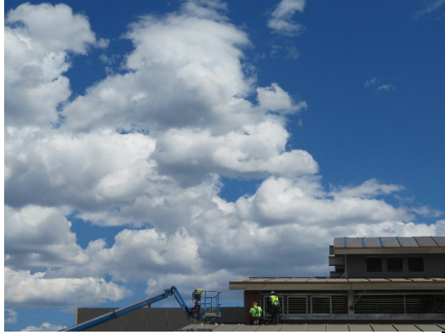
8/14/2019 – MTB Exterior Panels
