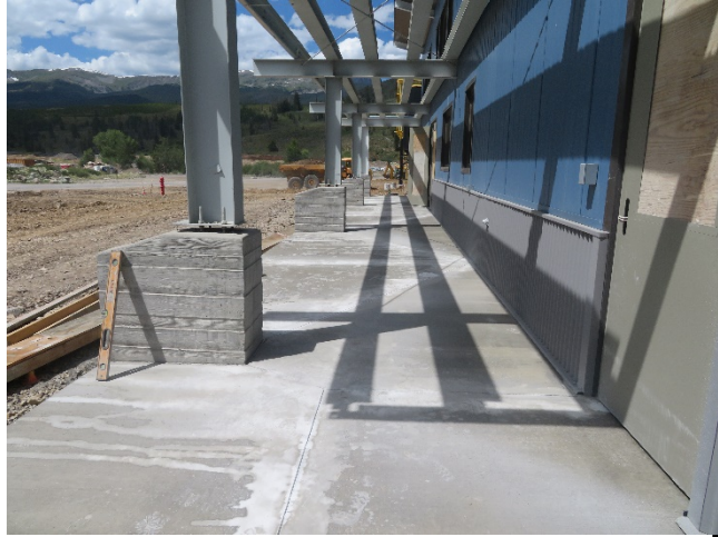
8/20/2019 – Administration Building Entry Concrete Sidewalk
