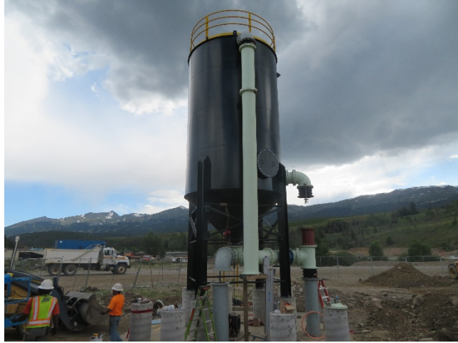
8/13/2019 - MTB Mixing Basin Fill Placement
