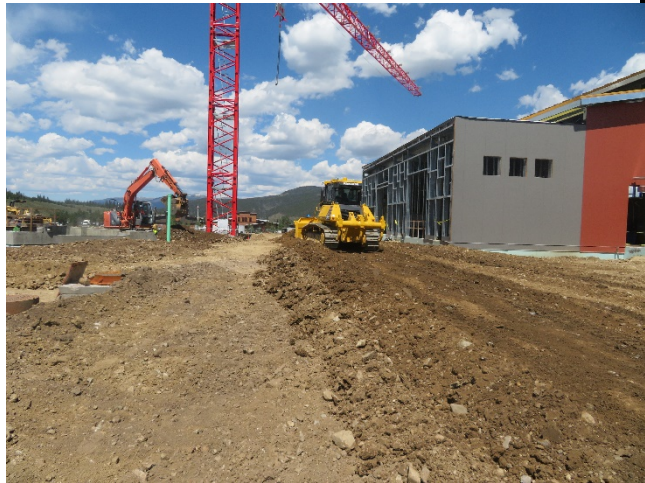
8/15/2019 – Backfill and Grading
