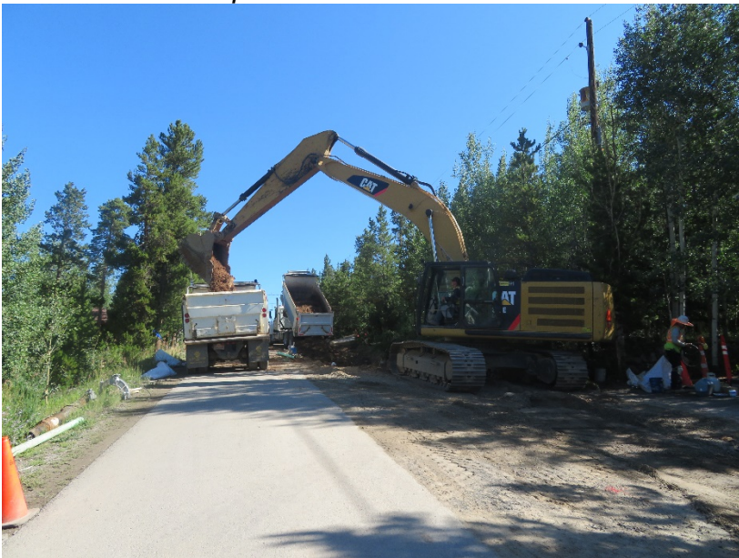
Finished Water Pipeline 8/15/2019
