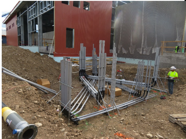
8/22/2019 – Emergency Generators Under Slab Conduits
