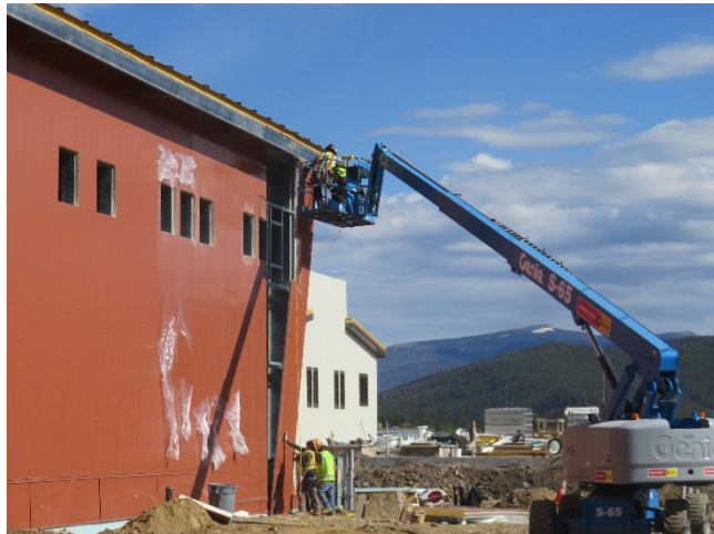
8/30/2019 – MTB Exterior Wall Panels
