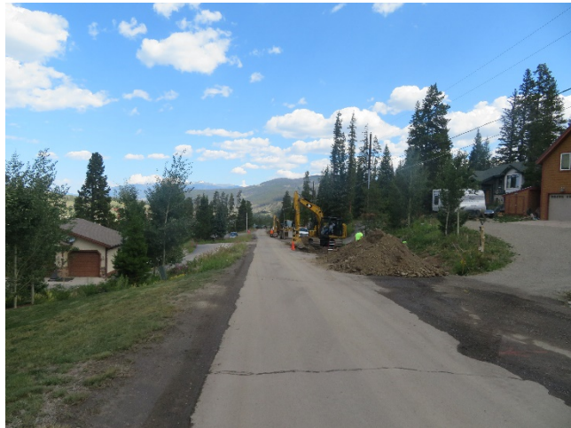
8/21/2019 – Fairview Blvd. Finished Water Pipeline
