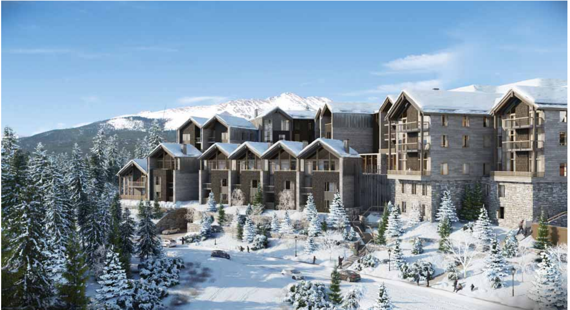
THESE IMAGES AND IMAGES CONTAINED HEREIN ARE AN ARTIST'S REPRESENTATION INTENDED FOR VISUALIZATION ONLY AND MAY NOT DEPICT ALL CONDITIONS ACCURATELY. REFER TO DRAWINGS FOR ACCURATE DESIGN.
