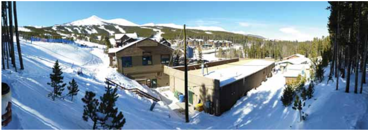
NORTH WESTERLY VIEW OF EXISTING ON SITE BUILDINGS
