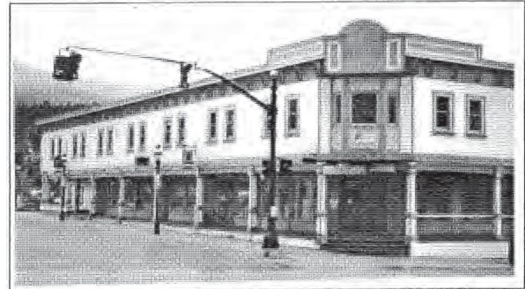
The Sterling Building is a fanciful imitative design built ca.1972. Although in scale with genuine historic buildings nearby, this newer building provides misleading information about the development of Breckenridge: the recessed arcade of the ground level is not typical of historic buildings in Breckenridge.
