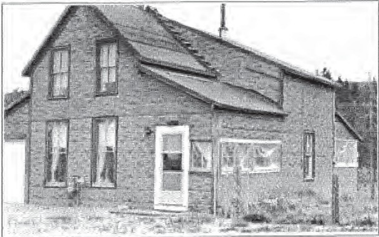
This photo of the Tillet House taken in 1978 shows an imitation brick siding that obscured the historic clapboard and diminished the integrity of the structure.
