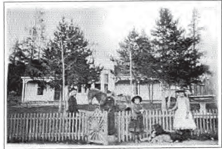
The C.A. Finding residence on North Main Street, as it appeared in the 1880's, contained some of the finer landscape features including an ornate wooden fence, plantings and a bird bath.
