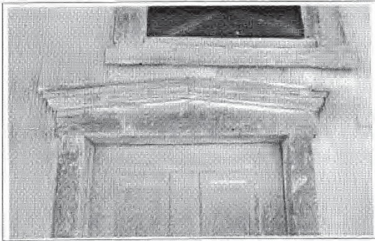
Preserve original ornament and detail of the facade.
