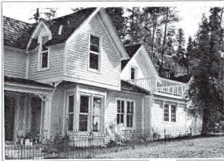
Additions should be compatible in size and scale. This addition, to the right, is distinguishable from the original building because of a joint in the wall plane.
