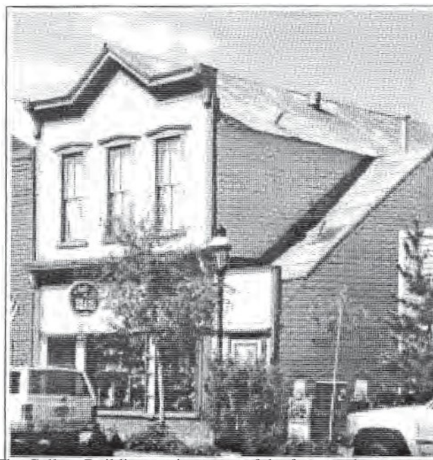
The Gallery Building retains many of the features that are typical of commercial buildings from the Camp Phase.
