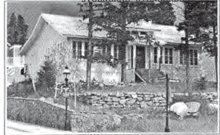
Native stone walls in a dry stack arrangement are encouraged, such as the upper wall in this photo. The lower wall is a moss rock veneer with mortar.
