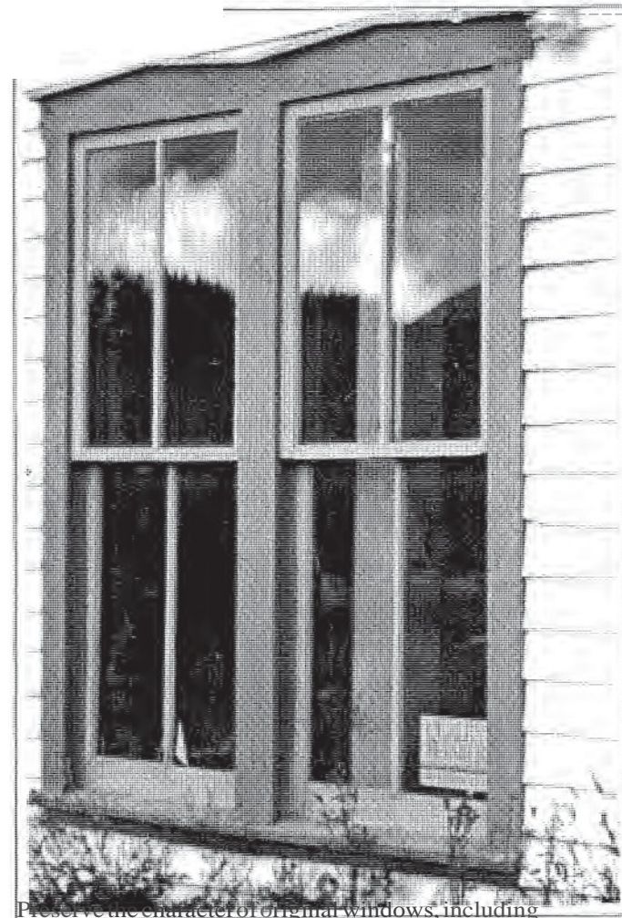
Preserve the character of original windows, including subdivisions. These give special character and scale to the building and the depth of the shadows they create helps to establish a sense of scale.
