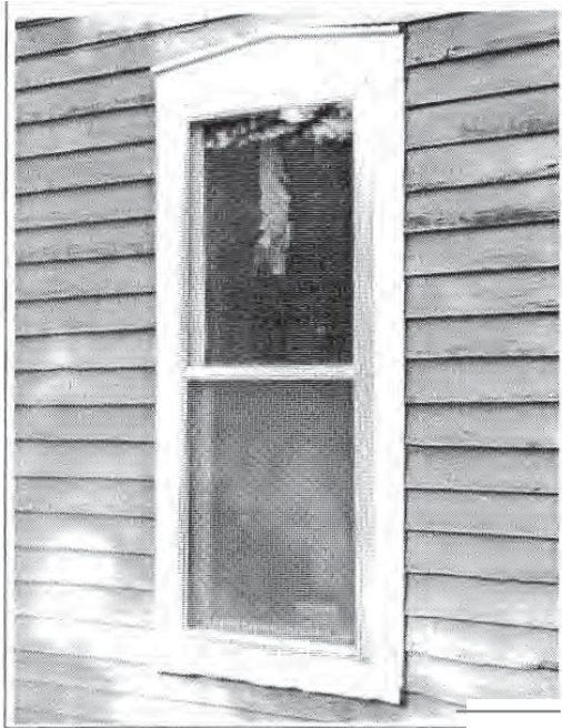
This exterior storm window matches the double hung arrangement of the original. Its appearance would be improved if it were painted, rather than raw aluminum.
