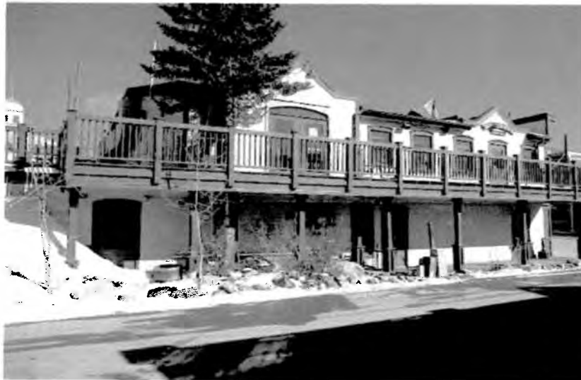
The West Southwest side of the Salt Creek Saloon. Solar collectors would be flush mounted to the roof behind and between the gables in this picture.
