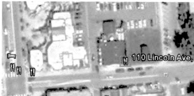
Salt Creek Saloon with Out Building in Rear as seen by Google Earth. The solar collectors will be on the left side of the roofs.
