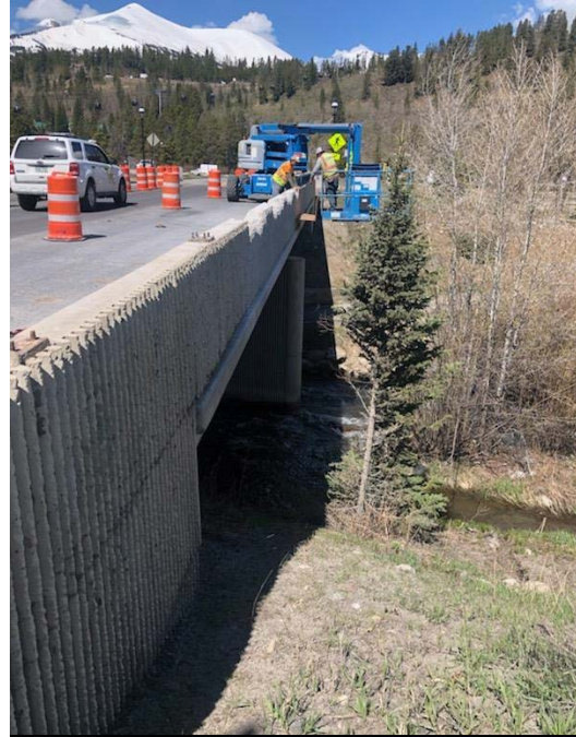
Work on the French Street Bridge.
