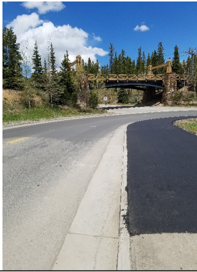
Ski Hill Road improvements.
