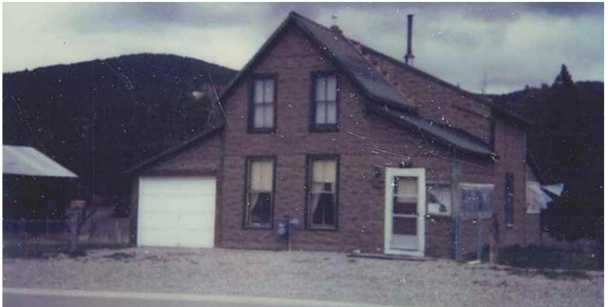
(Photo 4, above: Undated photograph from Town of Breckenridge property file)
