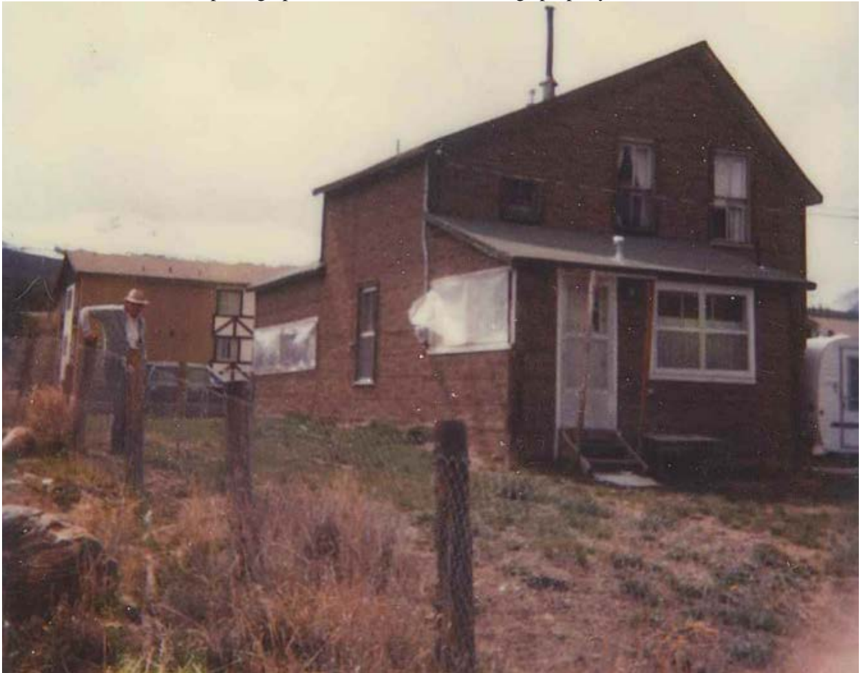
(Photo 6, above: Undated photograph from Town of Breckenridge property file)
