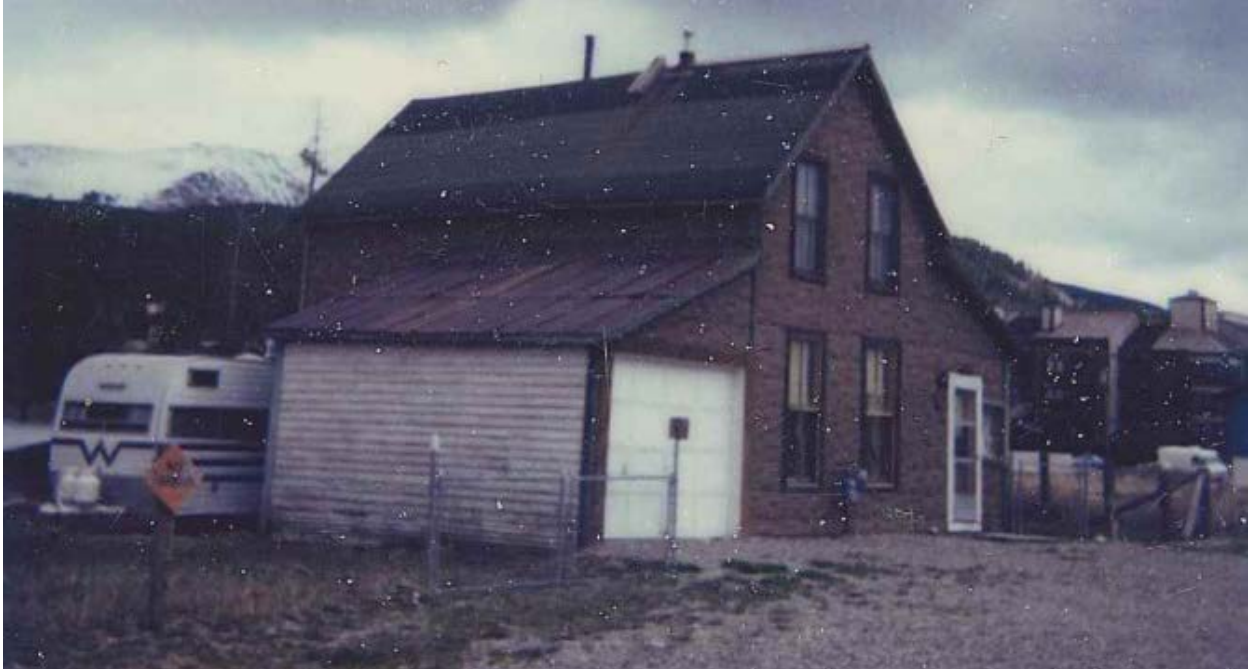
(Photo 5, above: Undated photograph from Town of Breckenridge property file)
