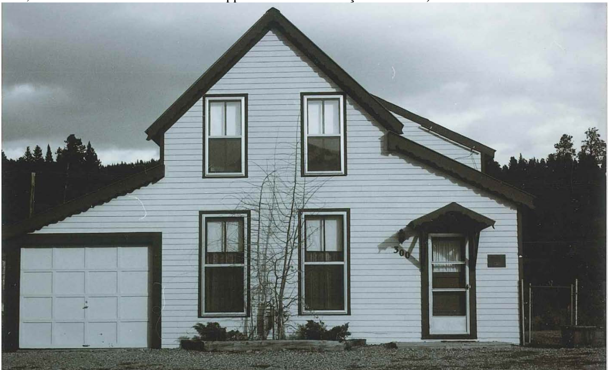
(Photo 8, above: Photo from Town of Breckenridge property file dated October, 1989.)
