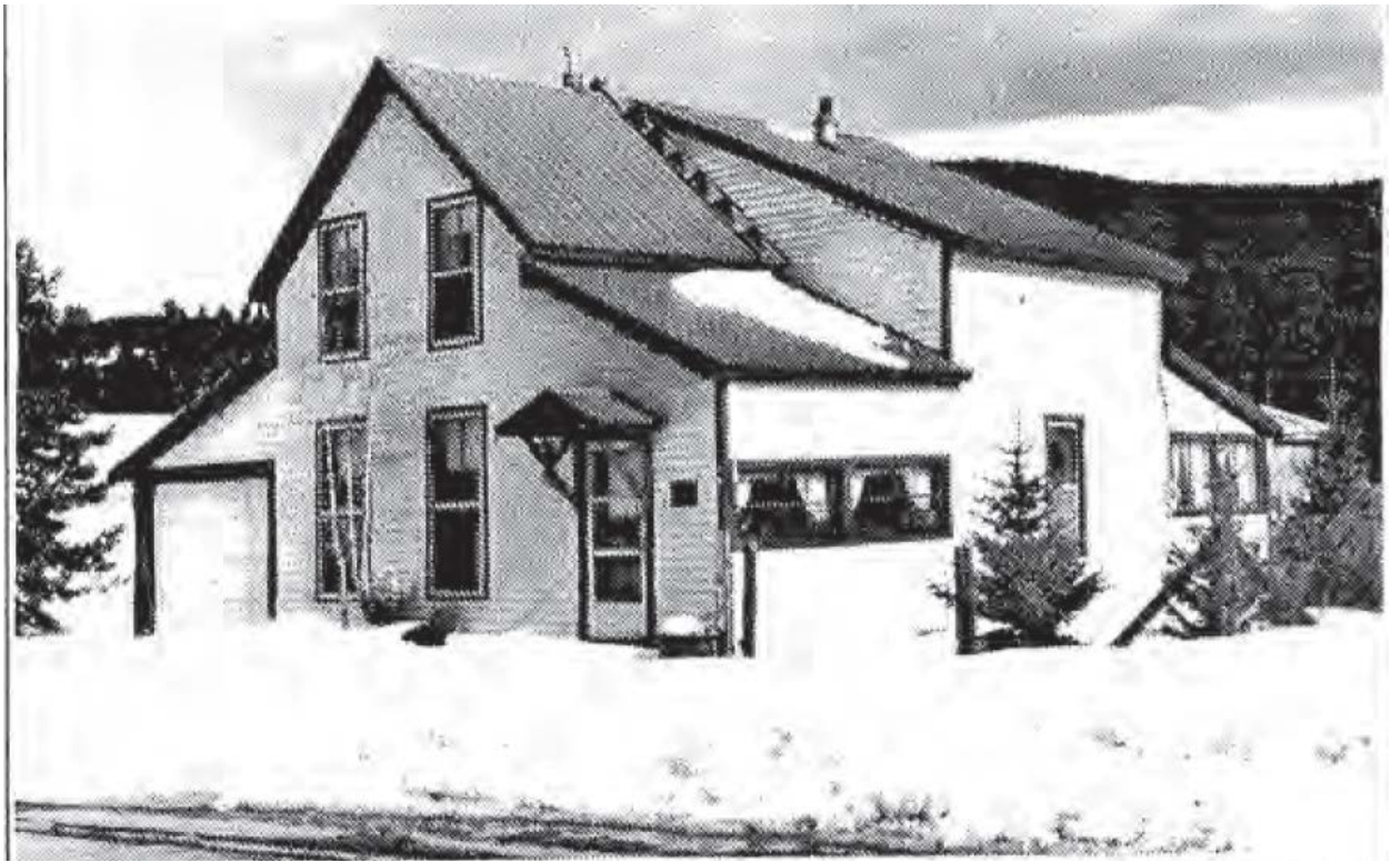
(Photo 7, above: Photo excerpt from page 29 of the Handbook of Design Standards, with caption “After rehabilitation, the historic material is visible and the historic integrity is enhanced” The window to the right of the front door has been removed, a small gabled cover added over the front door, and decorative wood trim detail appears on the front façade’s fascia.)
