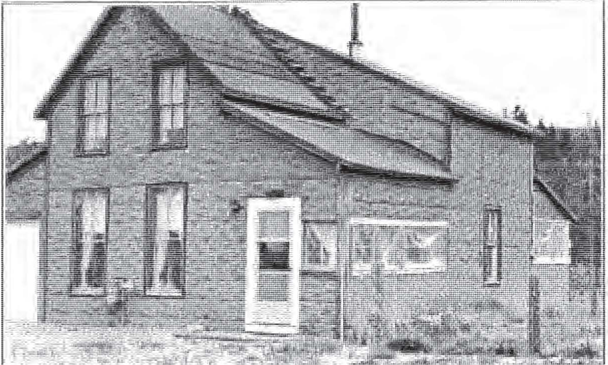
(Photo 3, above: Photo excerpt from page 29 of the Handbook of Design Standards, with caption “This photo of the Tillet House taken in 1978 shows an imitation brick siding that obscured the historic clapboard and diminished the integrity of the structure” An addition to the rear can be seen in the right hand portion of this photograph.)
