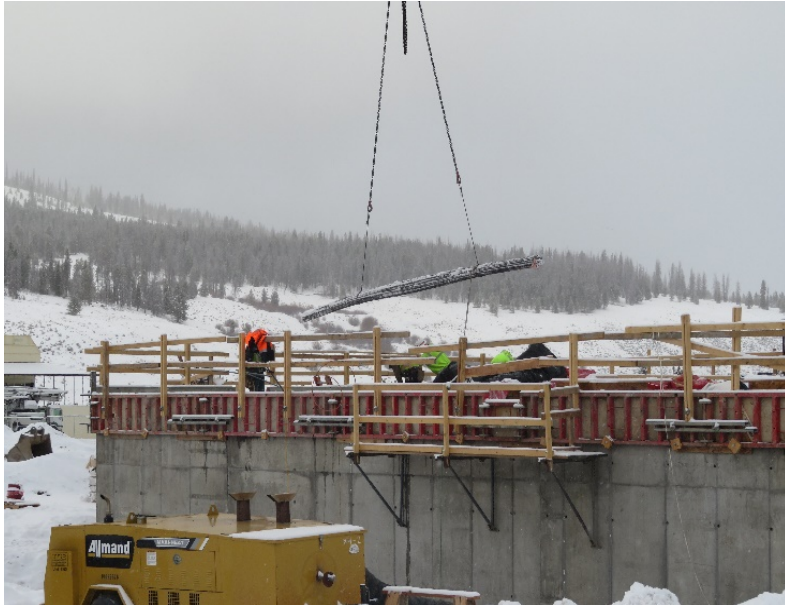
Finished Water Pump Station 11/02/2018
