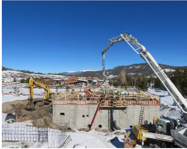
11/20/2018- Clearwell 1&2 Placing Concrete
