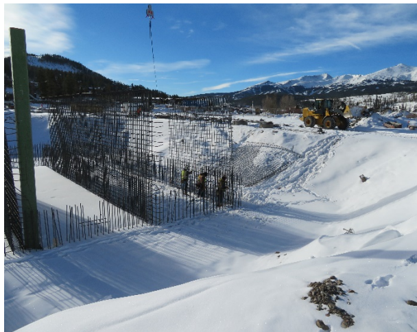
11/27/2018- Residuals Building Reinforcing Steel
