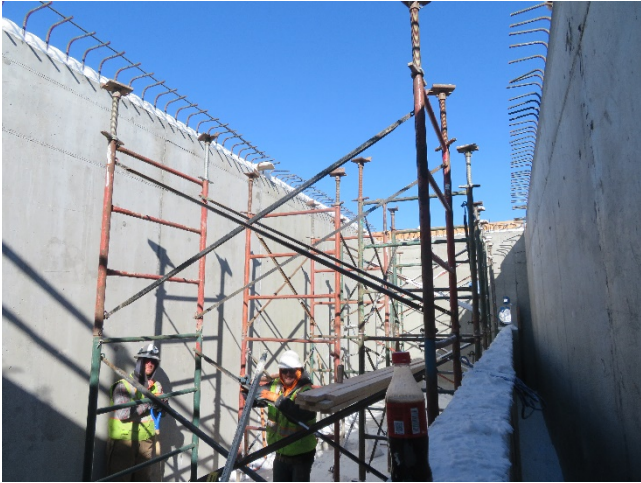
11/12/2018- Wet Well Shoring
