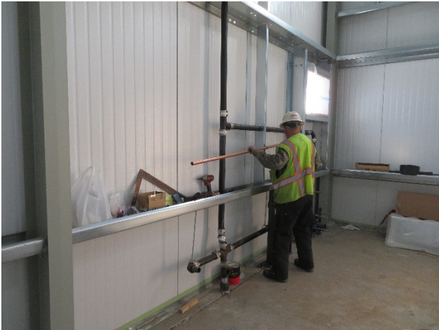
11/14/2018- Administration Building Plumbing
