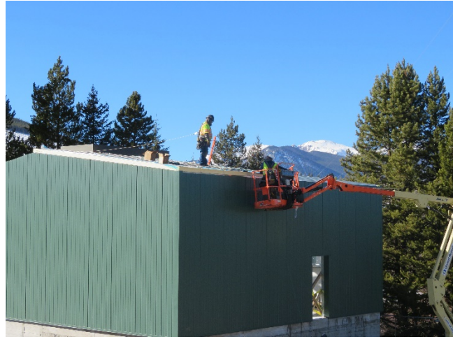
11/21/2018- RWPS Roof Panels
