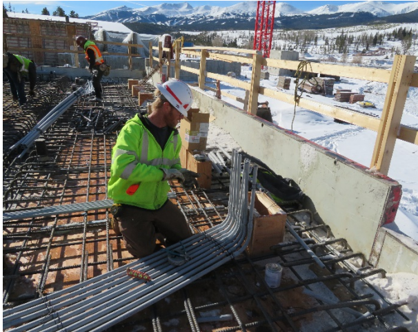
10/27/2018- Finished Water Pump Station In Slab Conduits
