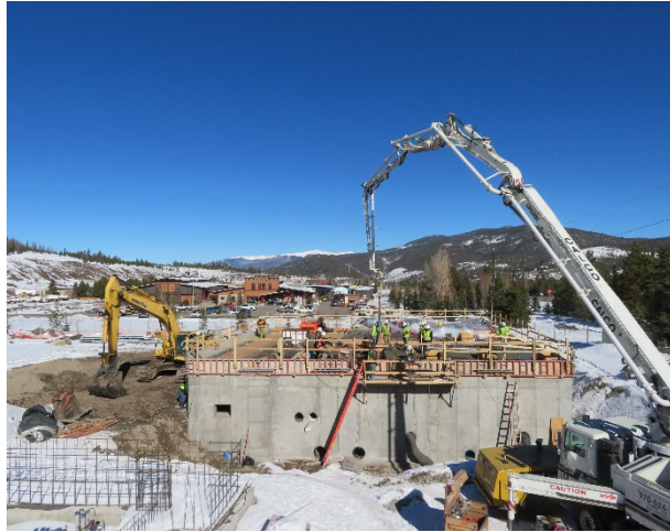
11/20/2018- Clearwell 1&2 Placing Concrete
