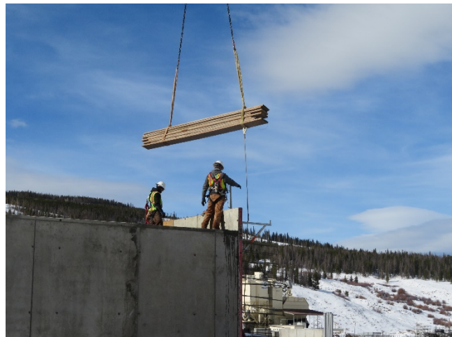
11/27/2018- Removing Planking at Filter Wall
