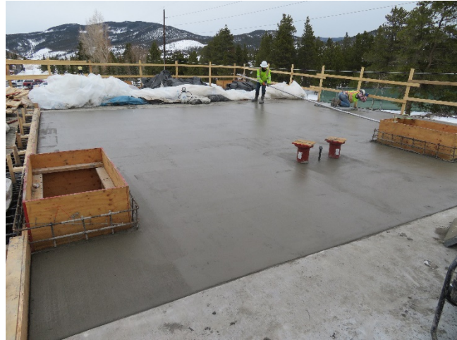
11/28/2018- Clearwell 1&2 Finishing Concrete
