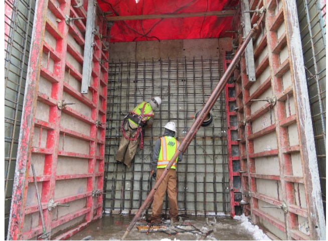
11/02/2018- Filter Wall Pipes
