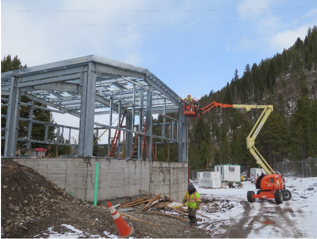
11/01/2018- Raw Water Pump Station Structural Steel Frame
