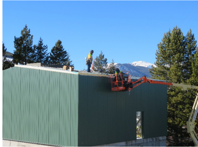
11/21/2018- RWPS Roof Panels
