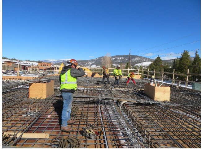
11/13/2018- Clearwell 1&2 Steel Reinforcing
