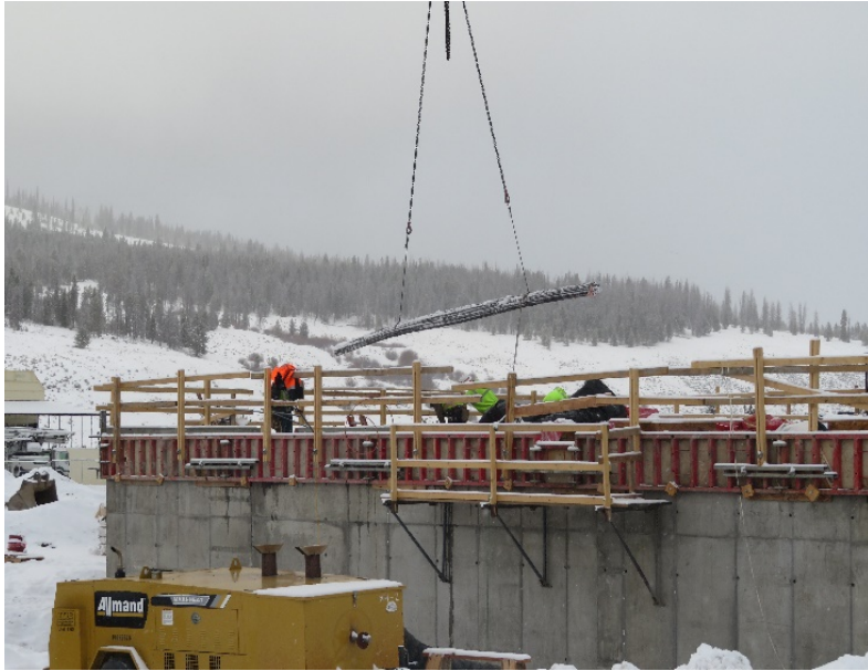
Finished Water Pump Station 11/02/2018
