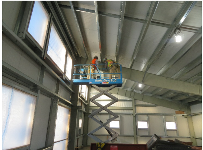
11/15/2018- Administration Building Painting
