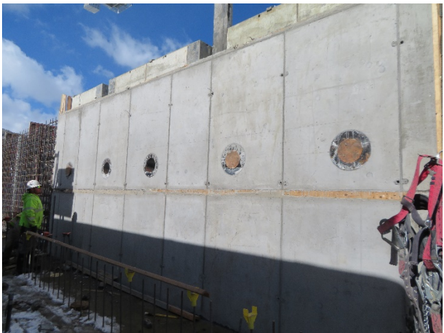
10/31/2018- Filters South Wall
