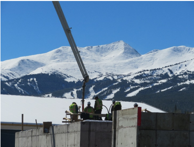
Treatment Plant Building Placing Concrete 10/16/2018
