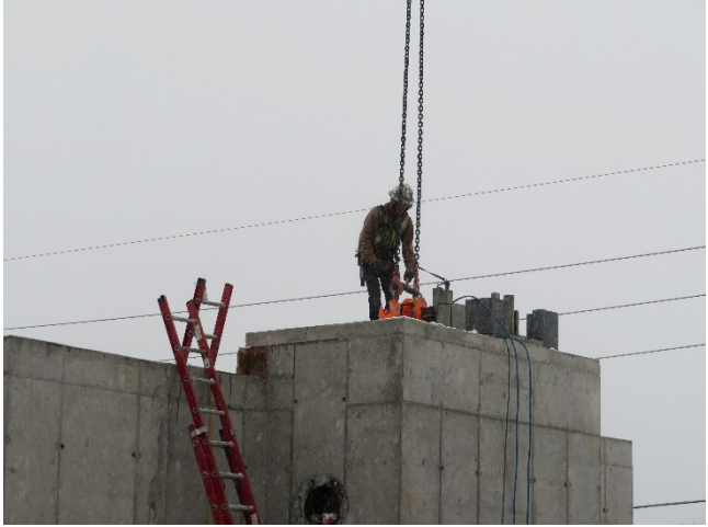
10/30/2018- Mixing Basins Removing Formwork
