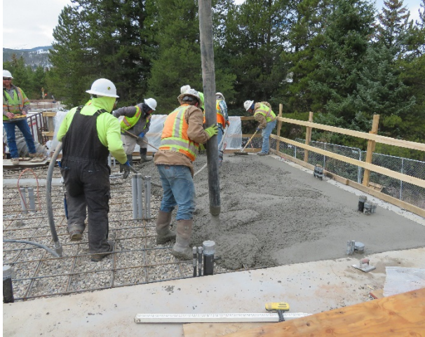
10/17/2018- Raw Water Pump Station Slab on Grade
