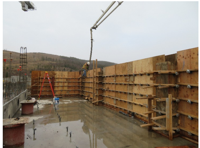
10/10/2018- Water Treatment Plant Placing
