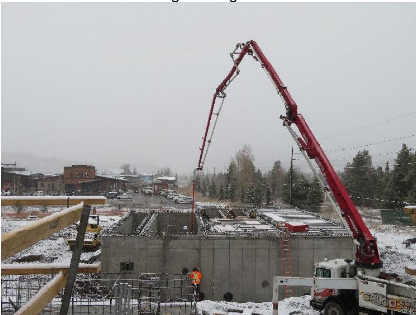
Clearwell Weir Wall Concrete Placing 10/30/2018
