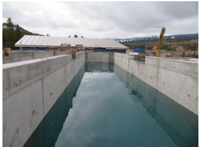
10/24/2018- Sedimentation Basin 3 Visual Leak Test
