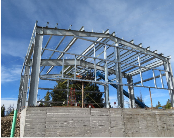
10/29/2018- Raw Water Pump Station Pre-Engineered Metal Building
