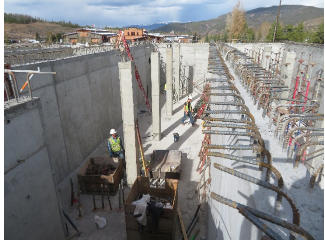
10/22/2018- Clearwell Baffle Wall Columns
