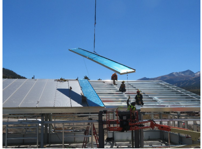
09/26/2018- Administration Building Roof Panels
