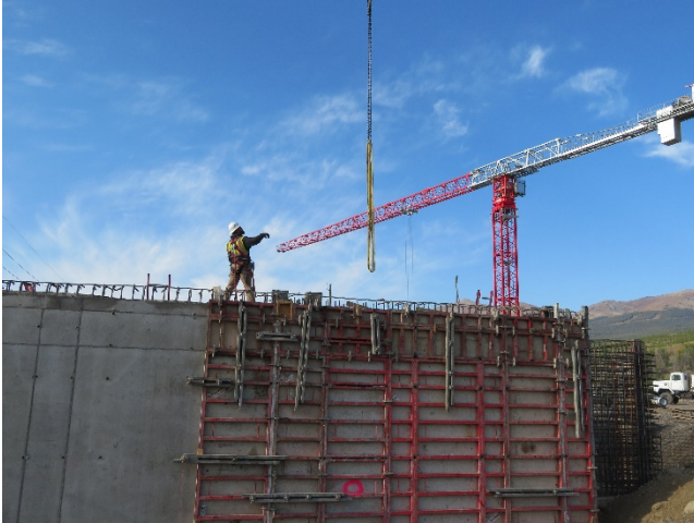
09/04/2018- Clearwell Removing Forms
