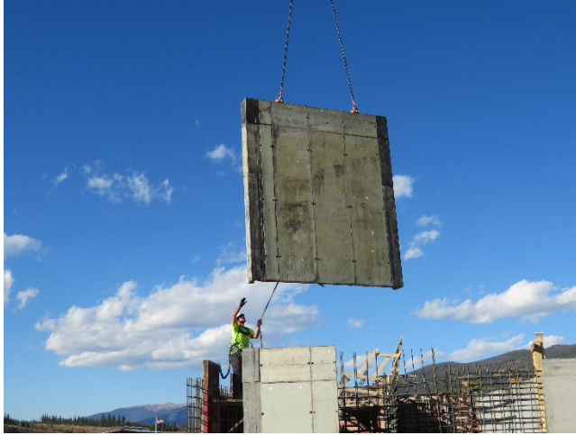
09/20/2018- Water Treatment Plant Gang Forms
