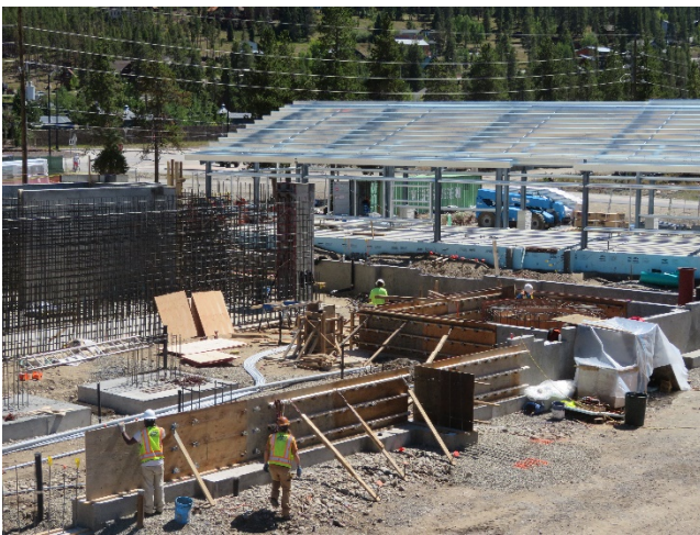
09/07/2018- Water Treatment Plant Stem Walls
