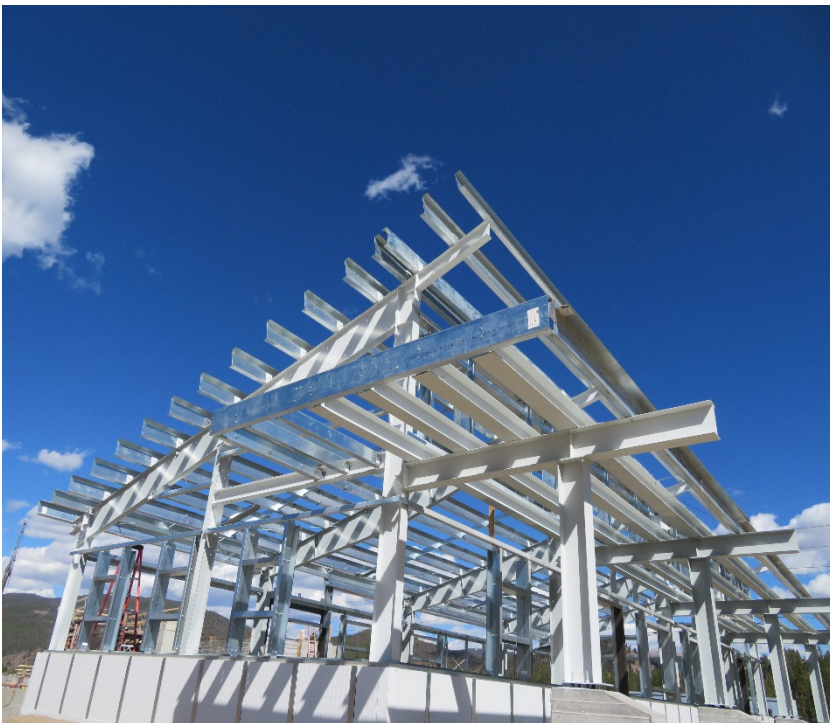
Administration Building Structural Steel Frame 09/20/2018
