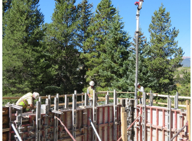
09/13/2018- Raw Water Pump Station Electrical Area Stem Wall Concrete Placing
