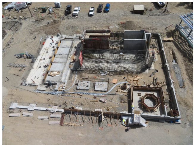
09/10/2018- Water Treatment Building from tower crane
