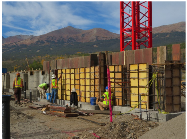
09/19/2018- Water Treatment Plant Stem Wall Formwork
