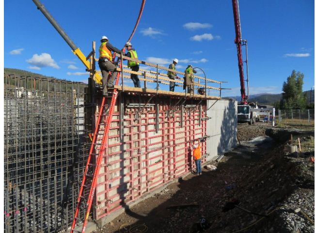
09/06/2018- Clearwell Placing Concrete
