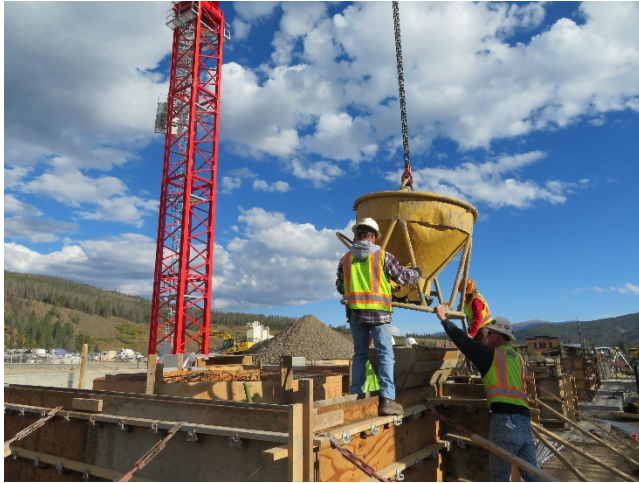
09/11/2018- WTP Placing PACL Containment Walls
