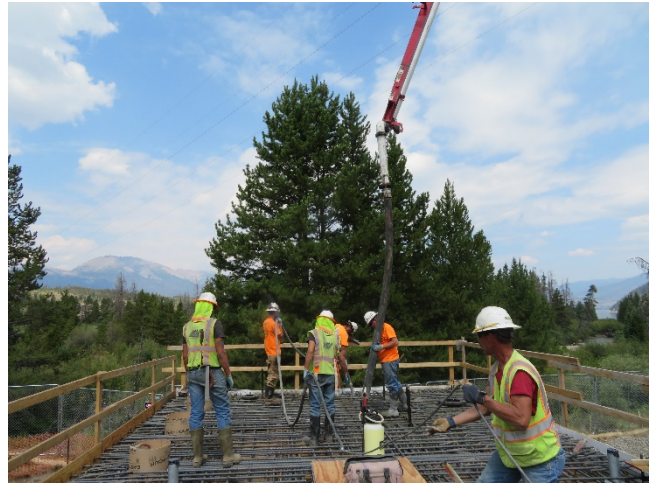
08/16/2018- Raw Water Pump Station Deck Concrete Placing
