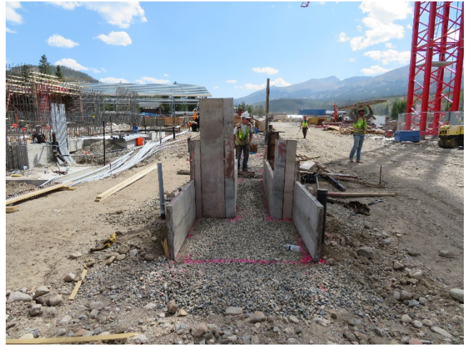
08/28/2018- West Stem Wall Footing
