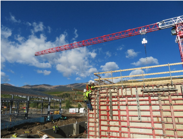
08/27/2018- Water Treatment Plant Gang Forms
