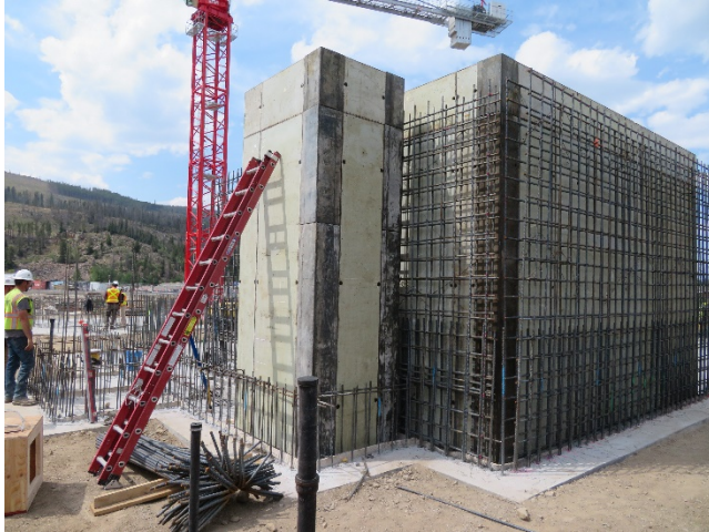
08/15/2018- Influent Channel Sedimentation Basin Wall Formwork
