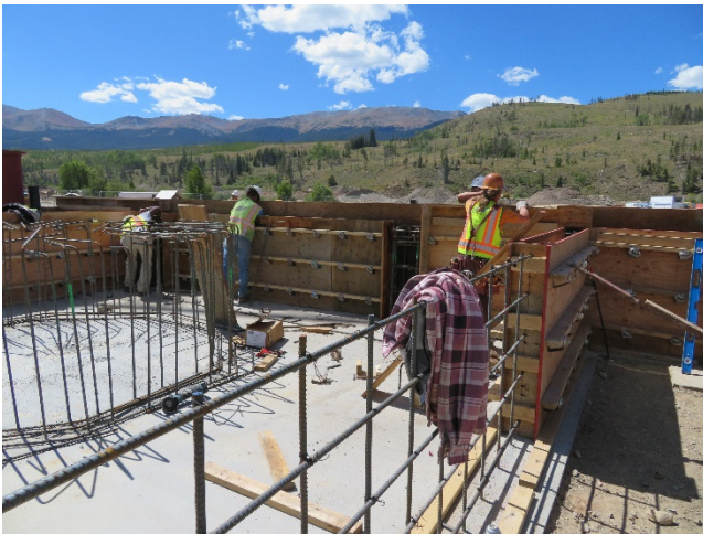
08/29/2018- Water Treatment Plant Stem Walls Formwork
