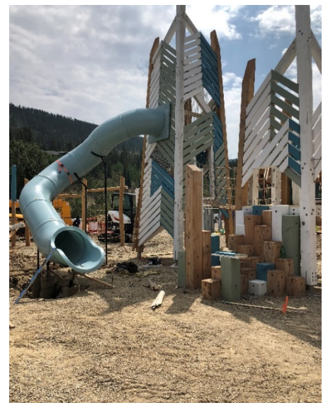
The installation of the playground equipment was recently completed.
