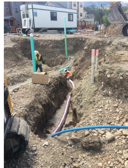
Sewer and water lines are being installed to the restroom building.
