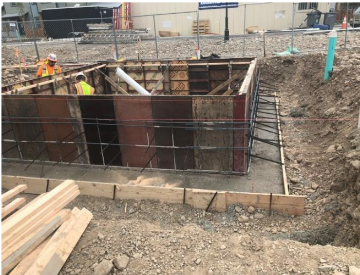
Foundations for the restroom/pavilion building are being formed.
