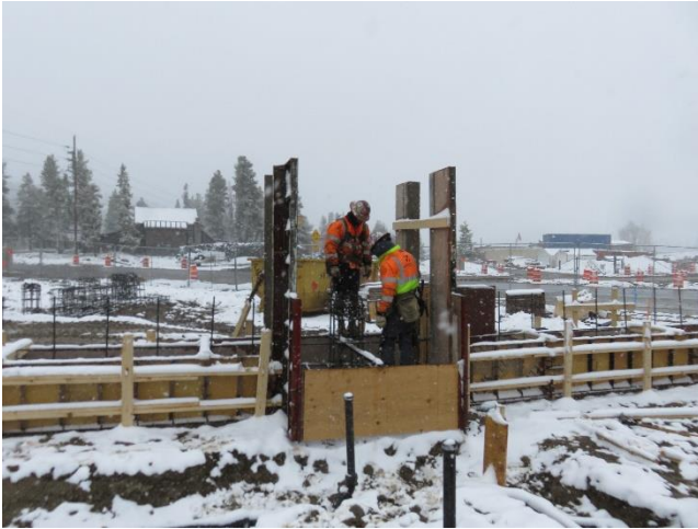
05/03/2018- Administration Building Formwork
