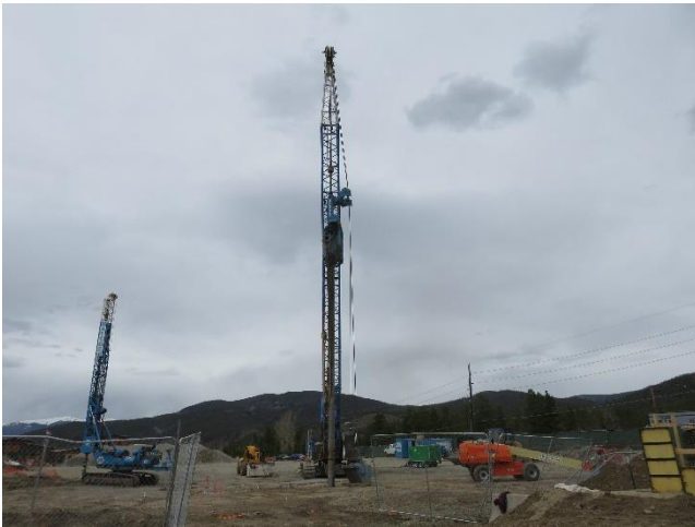
05/09/2018- Water Plant Vibro-Replacement
