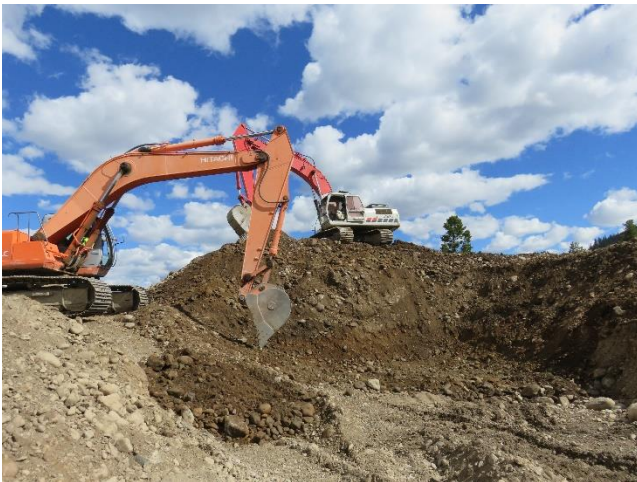
05/30/2018- Excavating Bore Launch Pit, 72 inch Sanitary Sewer
