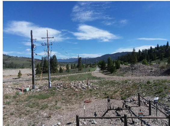
#7. Hwy 9 at Coyne Valley Road
