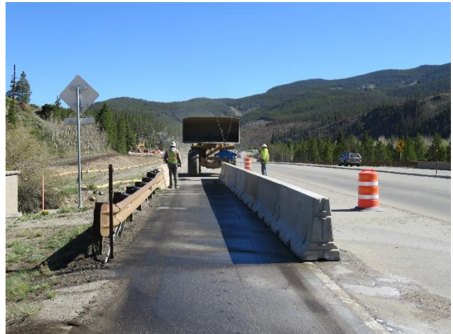
05/26/2018- Removing K-Rail at Swan Mountain Bridge
