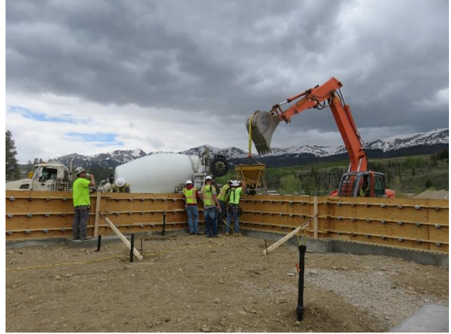
05/29/2018- Placing Concrete
