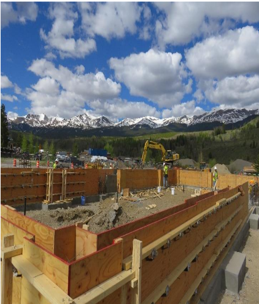
Administration Building Wall Formwork 5/30/2018
