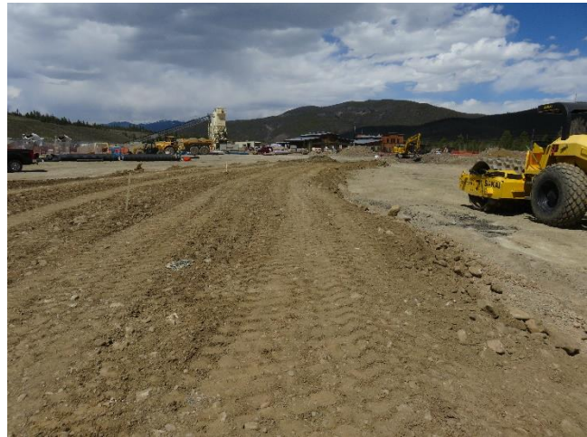
05/10/2018- New Alignment Stan Miller Road
