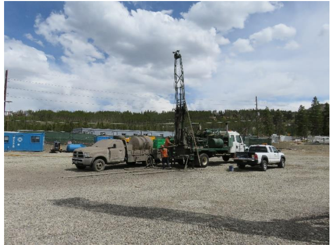
05/21/2018- Standard penetration test Drilling
