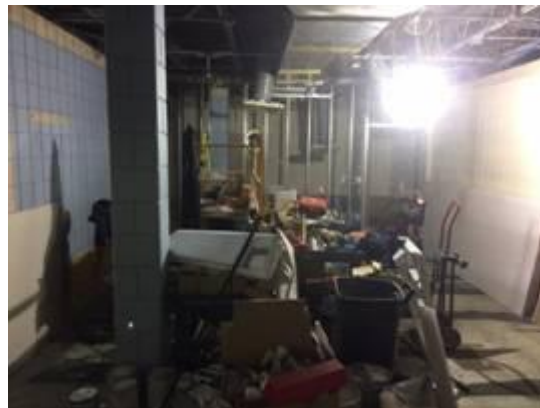
Downstairs Conference Room Construction
