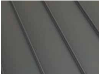
ROOF/FASICA AT FLAT ROOF METAL-BERRIDGE-STANDING SEAM-'SLATE GREY'
