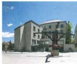
EXISTING PHOTO OF WEST ELEVATION
