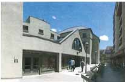
EXISTING PHOTO FROM SOUTH WEST
