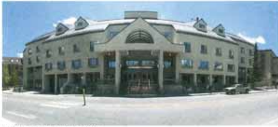
EXISTING PHOTO OF NORTH ELEVATION
