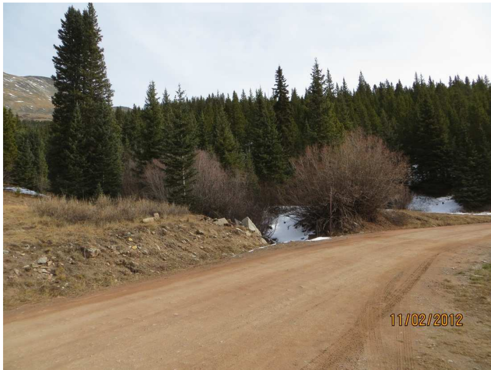
Photo 008, looking up road at drainage in basin 13.
