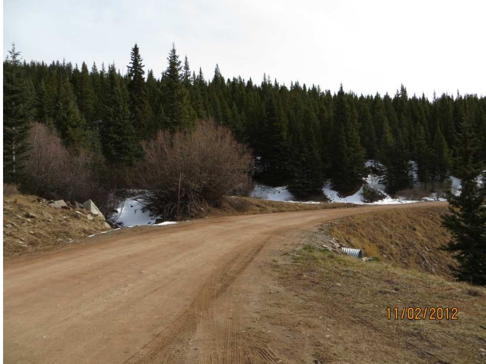
Photo 009, looking up road at drainage in basin 13.
