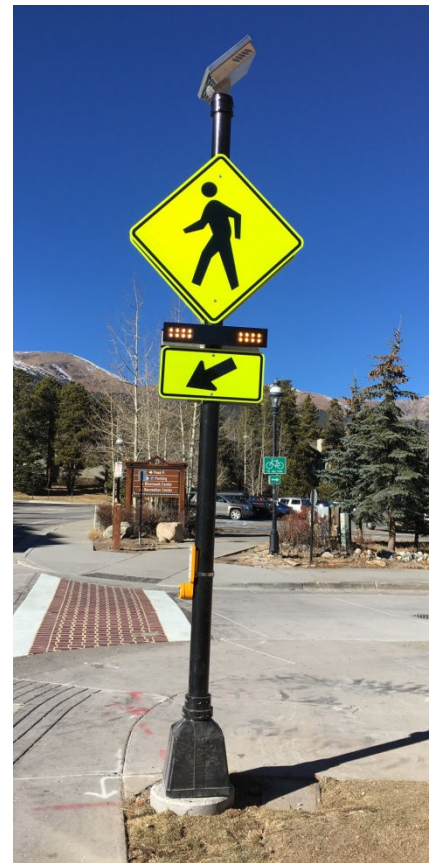
The new pedestrian flashing beacons installed at the crosswalk.
