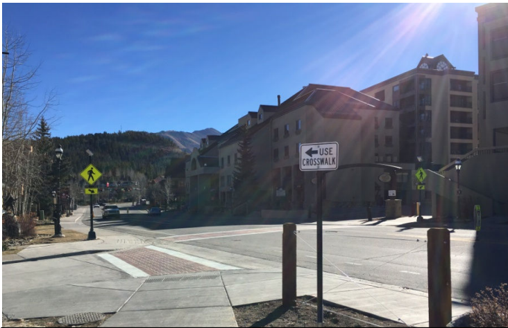
The new sidewalk, ADA ramp, fence, and sign were installed to direct pedestrians into the crosswalks.
