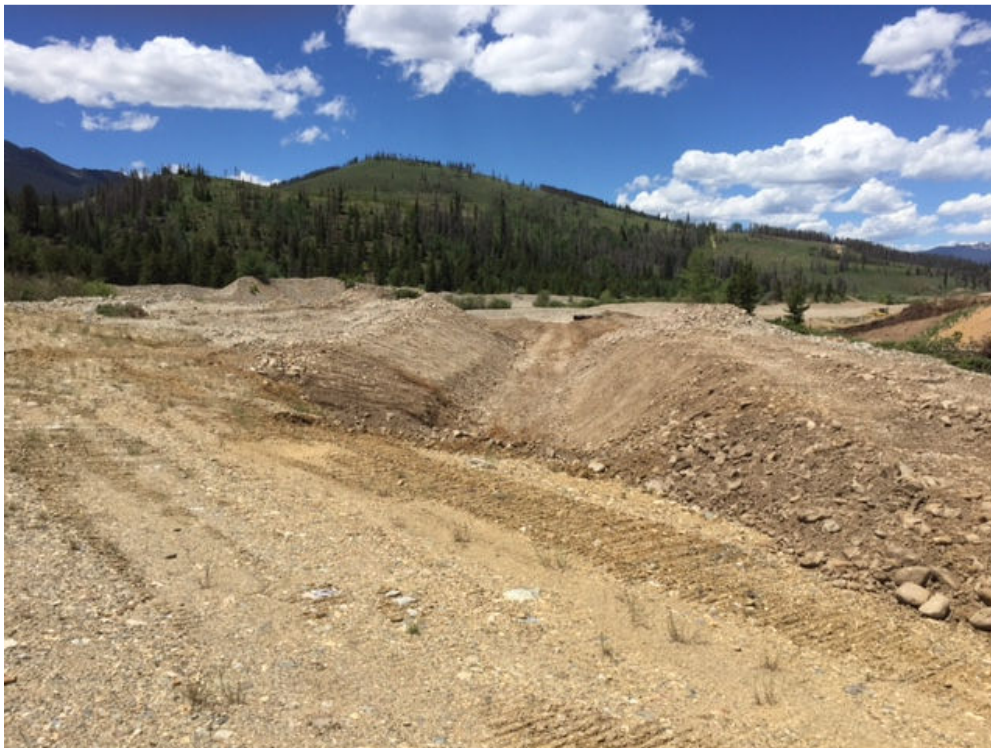
Blue River temporary river diversion construction north of Coyne
