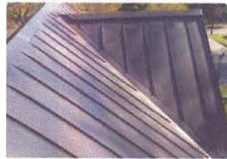
STANDING SEAM METAL ROOF ACCENT
