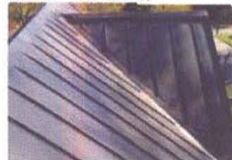
STANDING SEAM METAL ROOF ACCENT
