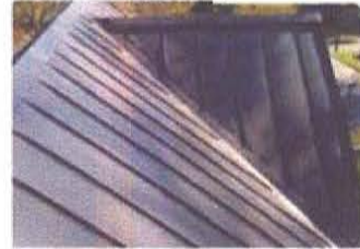
STANDING SEAM METAL ROOF ACCENT
