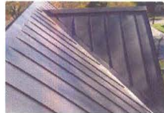
STANDING SEAM METAL ROOF ACCENT
