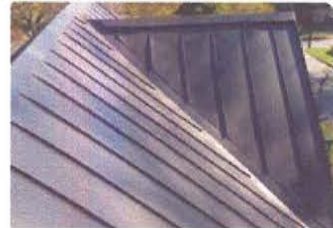
STANDING SEAM METAL ROOF ACCENT
