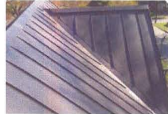
STANDING SEAM METAL ROOF ACCENT
