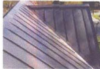
STANDING SEAM METAL ROOF ACCENT
