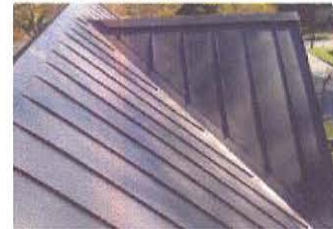
STANDING SEAM METAL ROOF ACCENT
