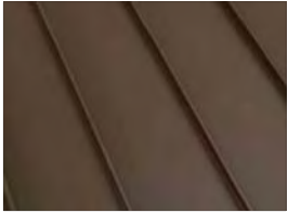
NEW STANDING SEAM METAL ROOF (CLASSIC METAL ROOFING SYSTEMS; COLOR: MUSTANG BROWN OR EQUAL)
