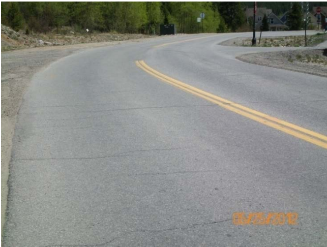
Transverse cracks at Reiling Rd at Rachel Lane
