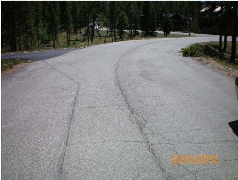
Block cracking with open cracks
