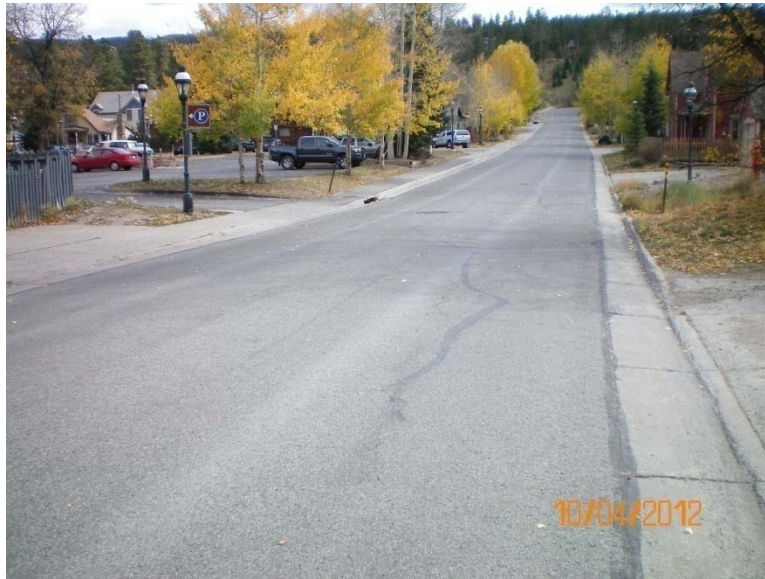
Widely spaced, sealed cracks
