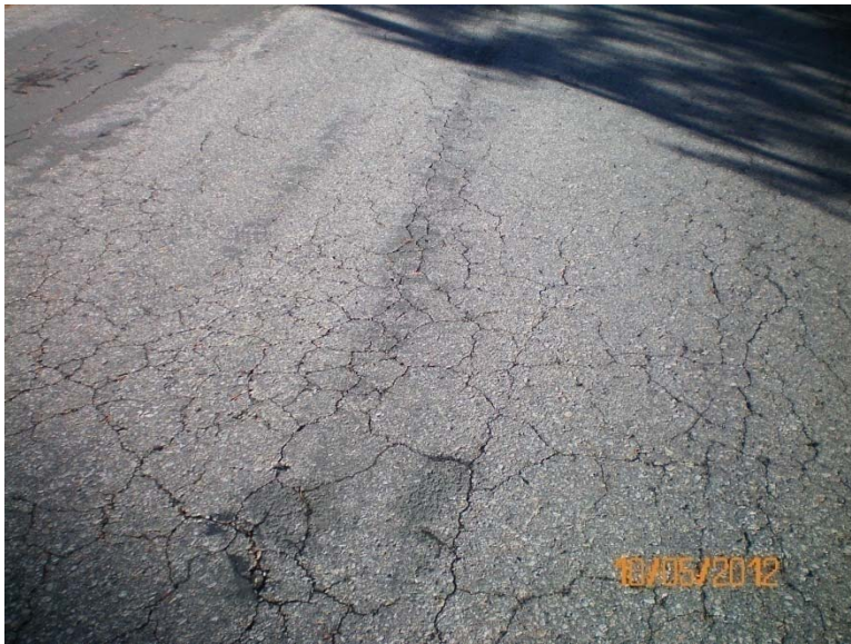
Block Cracking over 50%
