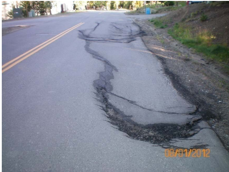
Slippage Cracks
