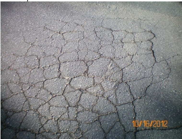
Alligator Cracks
