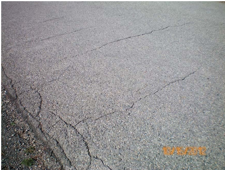
Longitudinal cracks near the edge
