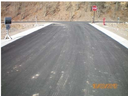
RATING 10 New Construction
