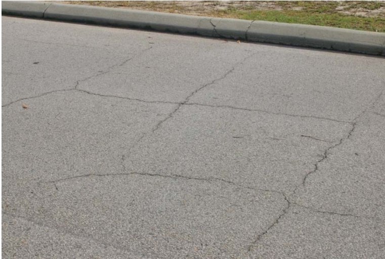
Block Cracking
