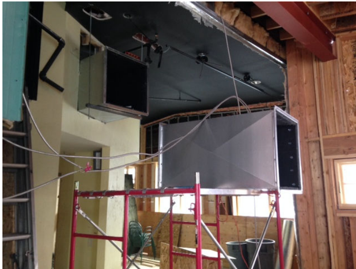
Ducting for the new HVAC system is being installed.
