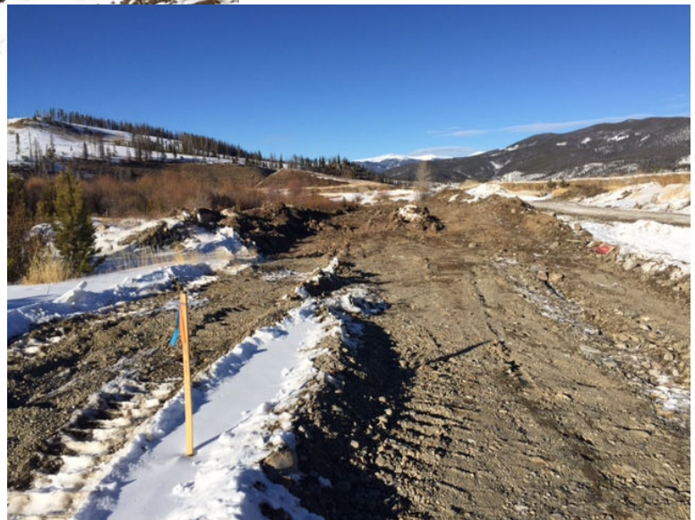
Rough grading of the temporary channel on the McCain site.
