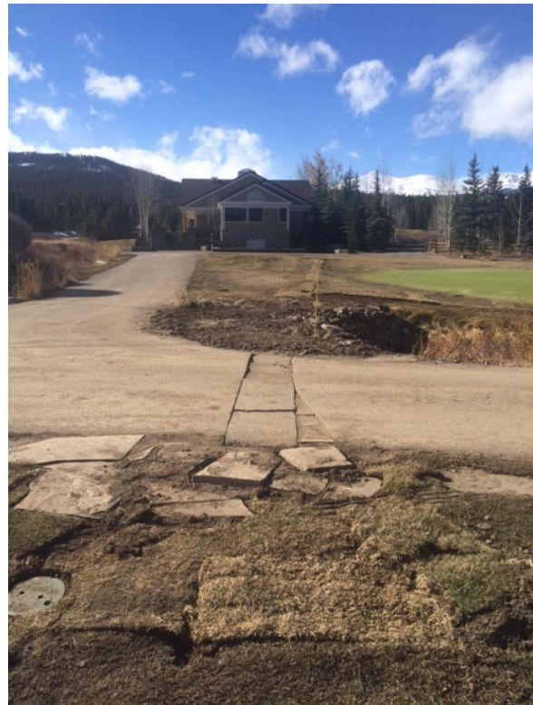
Work is finished and cleaned up.
