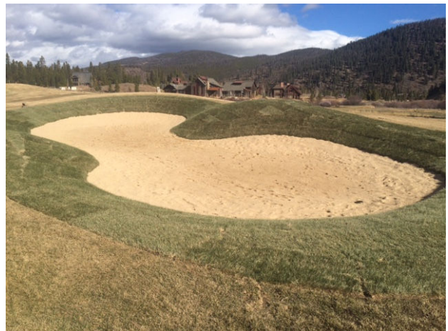
Sand and sod installed.
