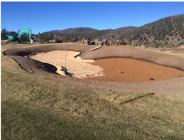
Liner finished, installing new sand.
