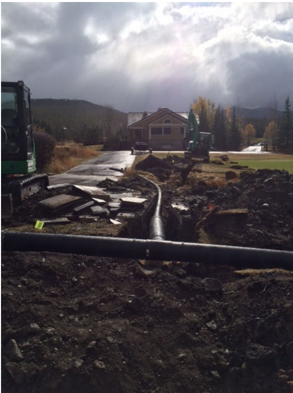
Installation of mainlines near the clubhouse
