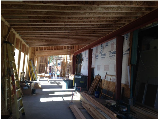
View looking west in the new lobby addition.
