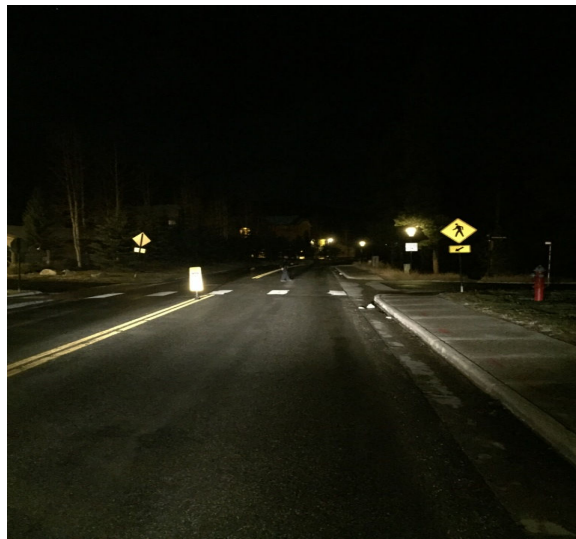
Facing North prior to crosswalk at 609 Airport Road, with headlights and person near crosswalk; 20 watt LED lamp bulbs
