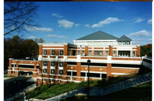
Figure 17: Examples of various façade materials used on parking structures
