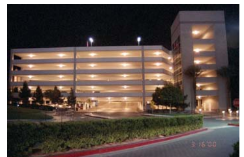
Figure 15: Example of Structure at Night
