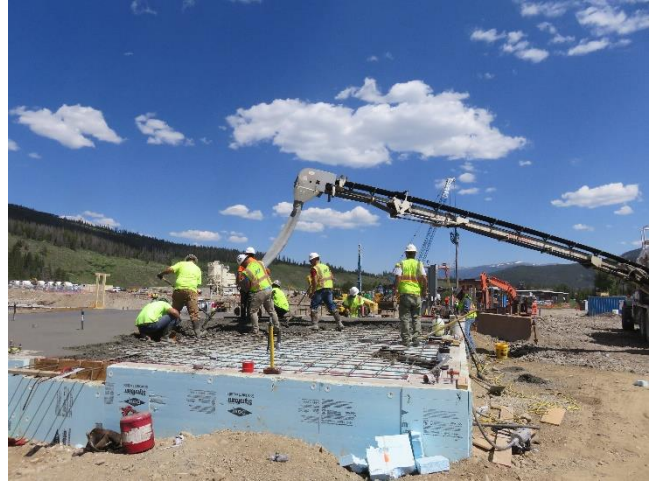
06/27/2018- Placing Concrete
