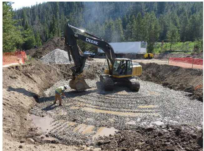
06/11/2018- Raw Water Pump Station Subgrade
