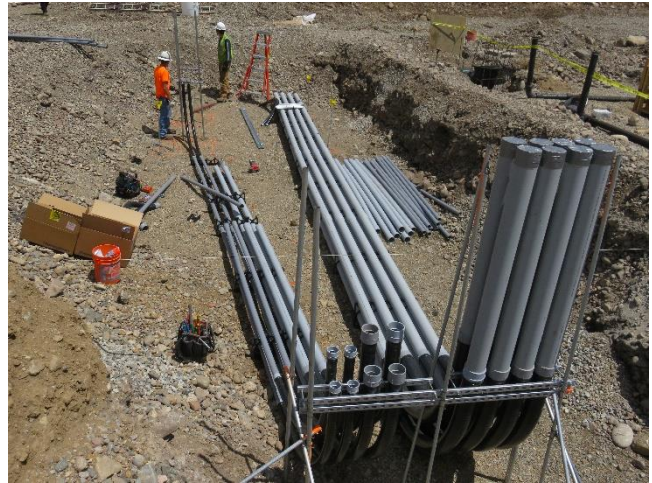
06/18/2018- Ductbank Generator to WTP
