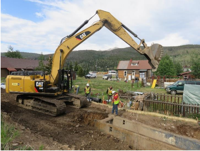
06/22/2018- Raw Water Pipeline
