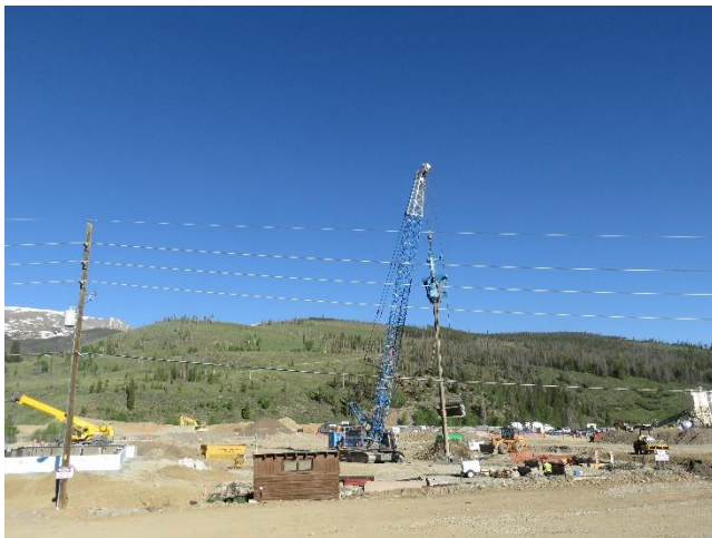
06/08/2018- Water Plant Vibro-Replacement
