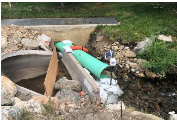
Upstream diversion of Sawmill Creek.
