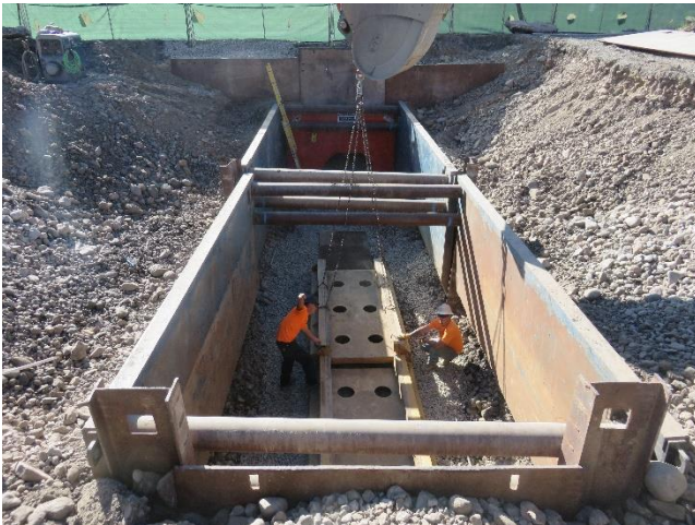
06/27/2018- State Highway 9 Finished Water Bore Launch Pit
