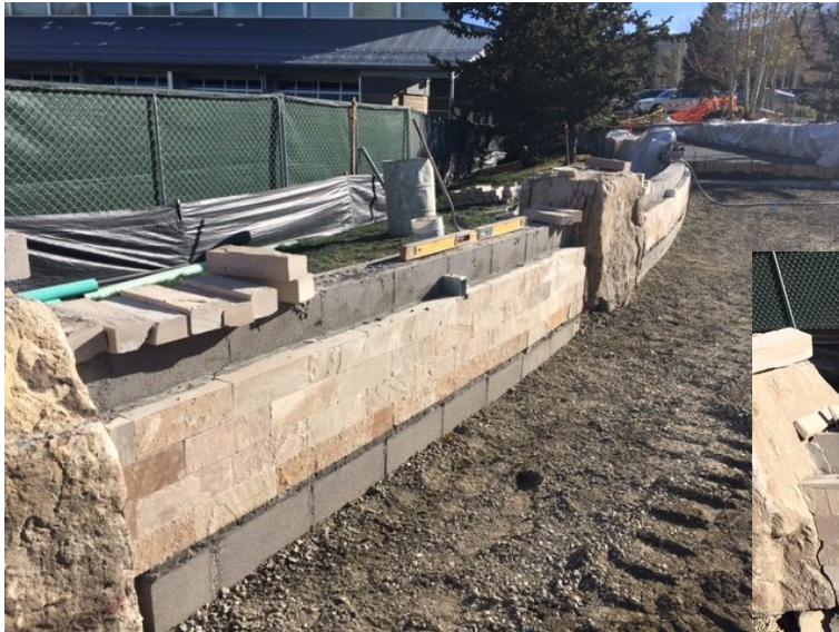
The new retaining walls are finished in a cut stone veneer.
